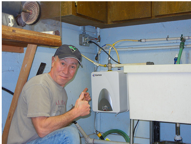
Frank with New Water Heater
